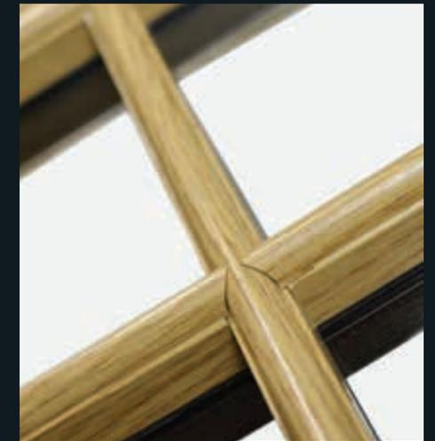
In order to meet modern building regulations and because we are not constrained by glass technology of the period, Residence 9 is made from complete pieces of glass where glazing bars are clad to the glass rather than making individual, small glass units. Internal spacer bars give the appearance of individual units, with the performance of a single, larger sealed unit.
